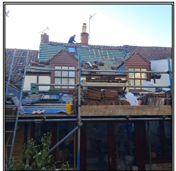
Re-tiling the house roof
